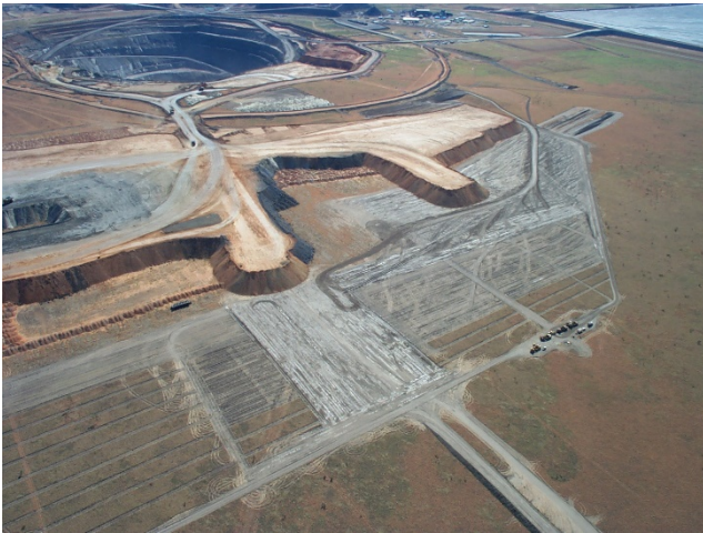
Figure 2. Aerial view of waste rock dump construction
