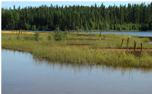
Figure 4. Revegetated dry soil cover over weathered pyrrhotite-rich Zn-Cu tailings in western Manitoba, Canada.
