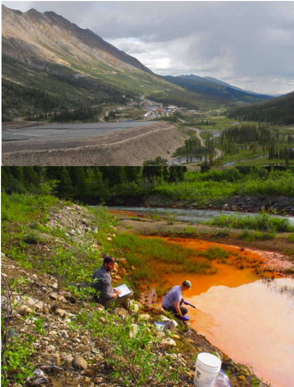
Figure 2. (top) view of Cantung site with tailings impoundment in foreground (photo E. Struzik). (bottom) oxidized tailings and iron-stained water near Flat River
