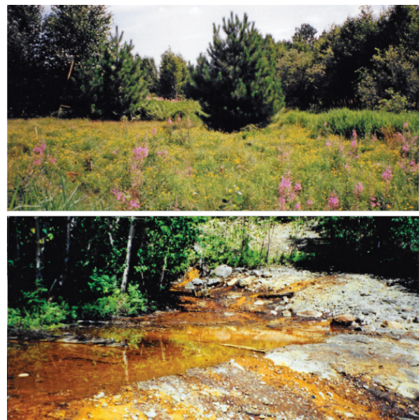
Figure 3. Revegetated dry soil cover over weathered pyrrhotite-bearing Ni-Cu tailings in central Ontario, Canada (top) and groundwater seepage at base of this tailings dam (bottom).
