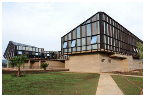
School of Mines and Metallurgy, Moanda, Gabon
